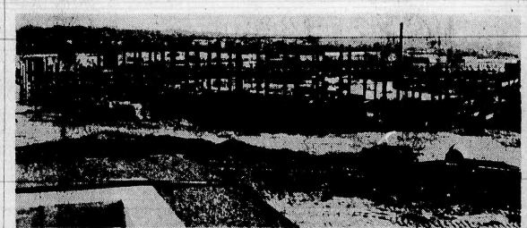
Picture above shows progress of the steel work for the new Clara Maass Memorial Hospital, which has now reached the third-story level. Workers have been somewhat hampered by the extreme cold of the past few days. Site of the new structure is near the Newark-Belleville-Bloomfield boulevards.
